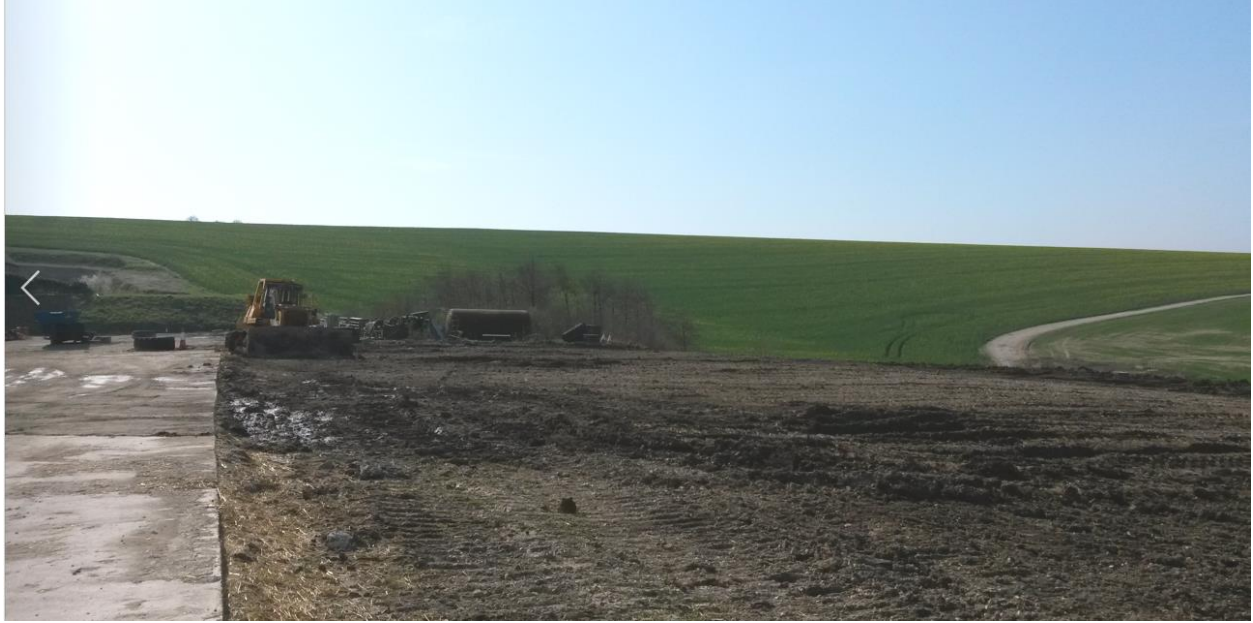
Profiled land to west of agricultural buildings looking towards Southwest
